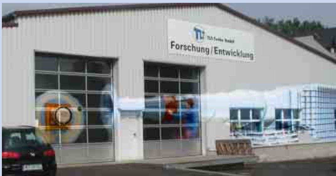
TLT R&D facilities
