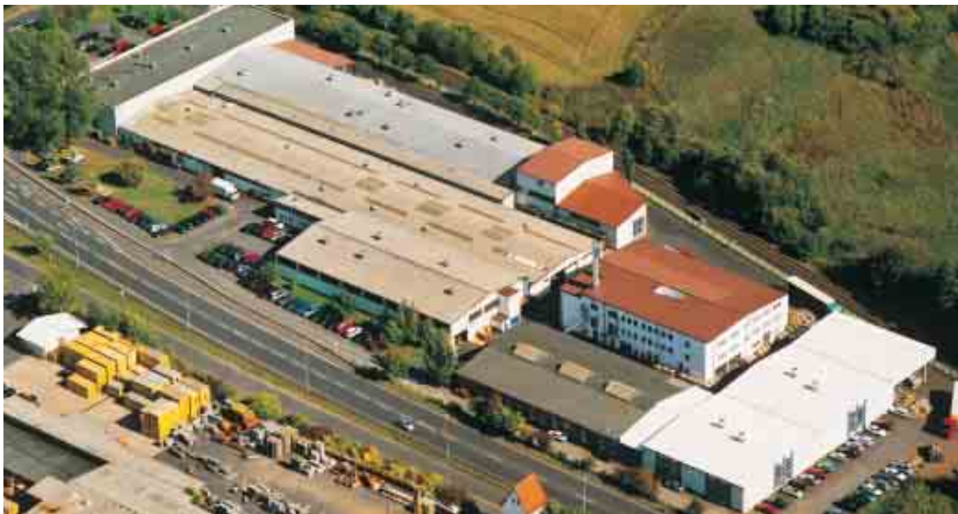
TLT standard fan production plant at Bad Hersfeld
