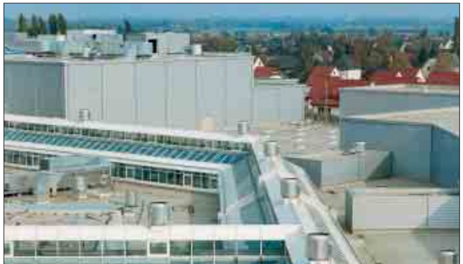
DVRF-H and BVD roof units on a shopping mall in Leipzig-Paunsdorf
