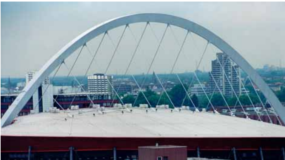
Roof-mounting smoke exhaust fans BVD 710 for 620°C–120 min. Cologne Arena
