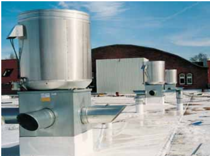
Roof-mounting smoke exhaust fans BVD 630/30-6 for 620°C - 120 Min. with stubs for admixture of ambient air (Berlin State Archives)
