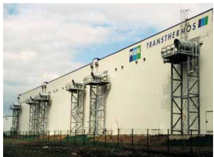
Axial smoke exhaust fan BVAXN 8/56/1120 for 600°C - 120 Min. with self-activating shutoff dampers and outlet duct with wire guard (Oyten refrigerating facility)
