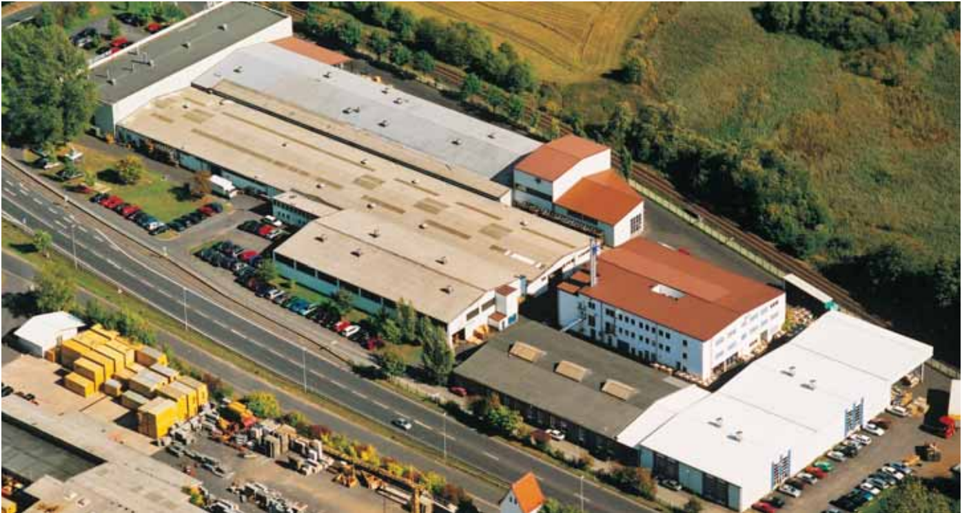
TLT standard fan production plant at Bad Hersfeld
