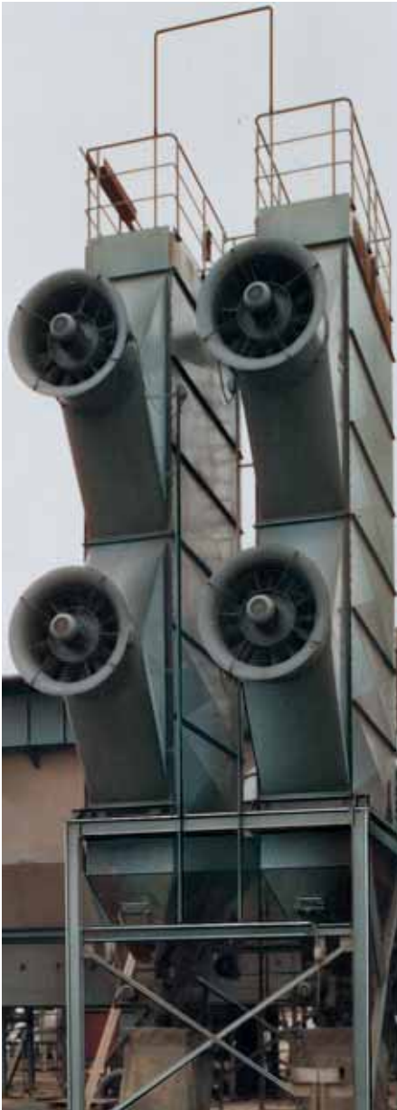
Forced-draught tubular heat exchangers equipped with AXN 12/56/100/M-S axial-flow fans (high-efficiency filtration)
